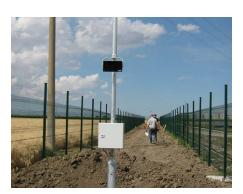
m length. Usually, one camera is able to cover about 60 m of the fence, so in total 30-40 cameras per plant are necessary to monitor the area. NETAVIS Observer, the professional video management platform known for its open and flexible software architecture, governs the video surveillance installations.
